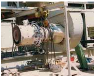
C40 engine being removed from package after breakdown
